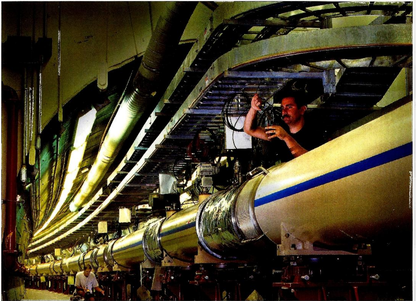
The RHIC heavy ion collider at Brookhaven. The Megascience nuclear physics working group recommends more co-ordination and collaboration to strengthen the worldwide effort in heavy ion collision physics.
